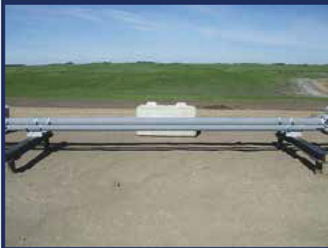
Pre-Build Pipe Stand Sliders
