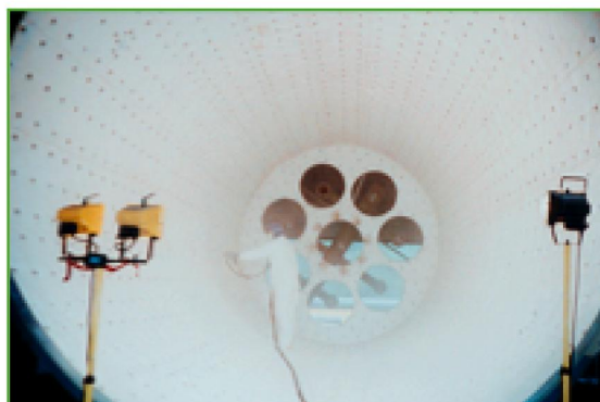
Ceramic Fiber Blanket Installation
