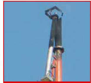
Competition's Wrecked Shroud and Flame Lick Damage
